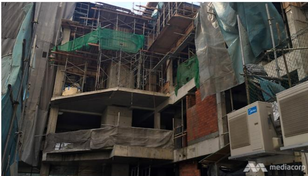
File photo of a construction site along Geylang Road without proper scaffolding and safety barricades in place. The construction company was issued a Stop-Work Order (SWO) of three weeks under new conditions imposed on May 12, 2016. (Photo: Loh Chuan Junn)
